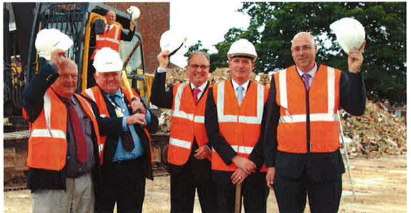
Town and Borough Officers and members at the start of the demolition
