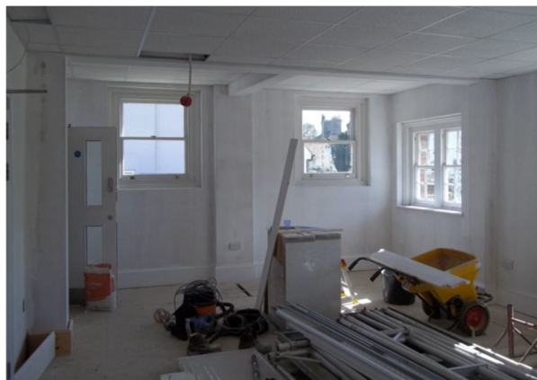
Suspended ceiling installed in office and decorating underway.
