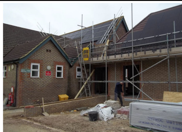
Solar panels being installed
