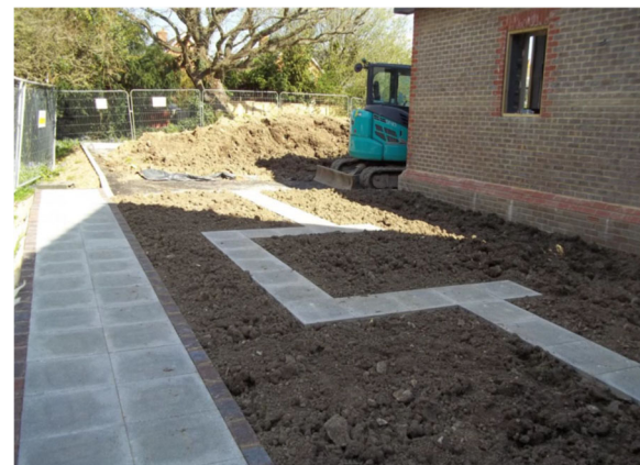
Soil inserted around paving to rear garden area
