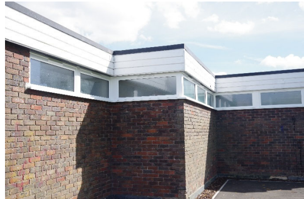
Innes Pavilion old windows replaced
